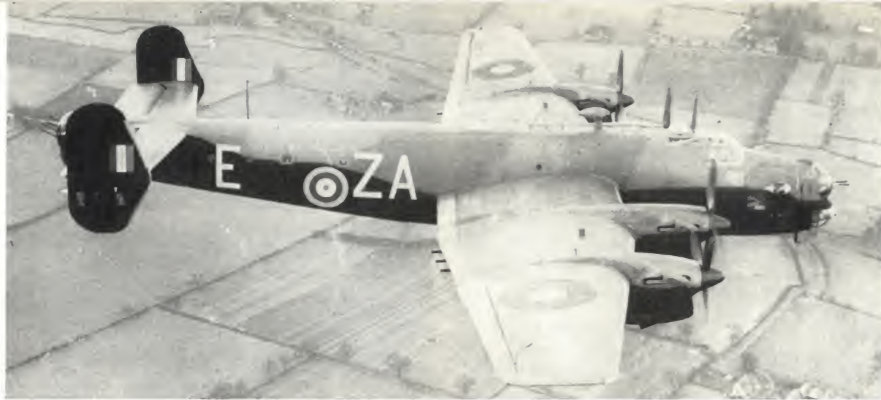
An unusual Halifax was L9619, a Mk II seen here without a dorsal turret and in the hands of 10 Sqn. She joined 10 Sqn in November 1941 and crashed on the night of February 15/16. Note the camouflage patterning and an almost invisible red serial ahead of the 'E' on the upper surface colouring (Imperial War Museum).
